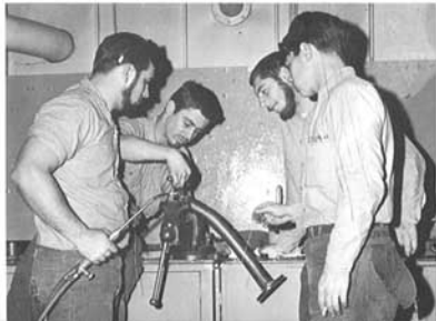
Beiter and Macchia watch (above) as Zielinski sketches cut to be made in sheet metal. (right) DC's repair a lub oil line for B-3 generator by brazing.
